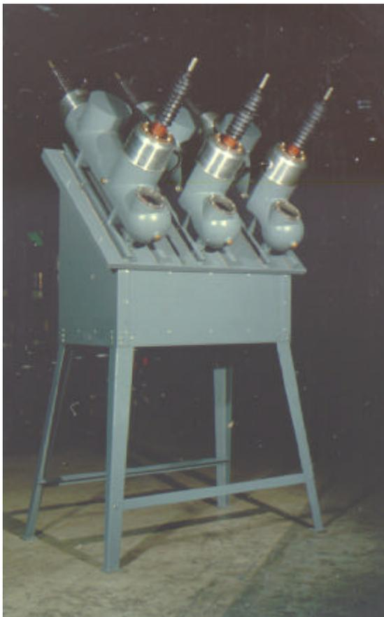
*Figure 1.1 An OX 36kV outdoor circuit breaker. This is a typical piece of outdoor Medium Voltage switchgear. Inside each tank is one V8 type vacuum interrupter rated at 36kV; 25kA;1250A. Circuit breakers are also housed indoors in substations and also used for special applications. For example the same type of vacuum interrupter is fitted in a different single phase 25kV circuit breaker mounted on the roof of the Eurostar train, just behind the pantograph.*
