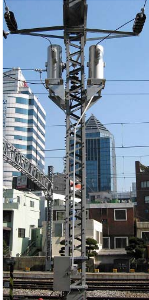
Figure 9. Two SDR single phase circuit breakers for railway applications. This uses the basic design and many components of the VOX rearranged in a new stainless steel tank to give a compact, simple, single phase, catenary mounted, circuit breaker which can be mounted in several orientations depending on requirements.
