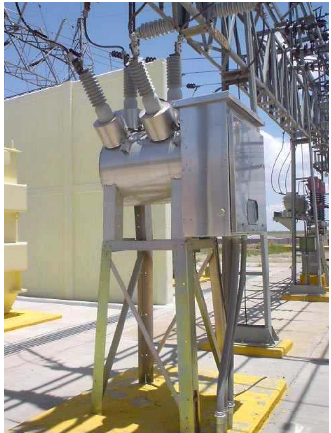
Figure 4. VOX circuit breaker c.2001. All three interrupters (VG type rated at 38kV;25kA;1250A) are now housed inside a single stainless steel tank containing SF 6 .
